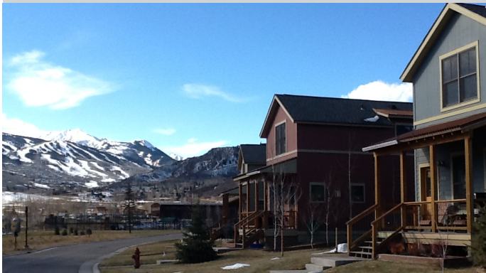
Rodeo Place, Affordable Housing in Snowmass Village, Colorado
