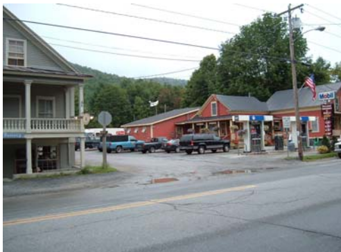
The Parsonage Lane-VT 100 intersection lacks definition. There is a continuous curb-cut along Parsonage Lane to the Village Grocery.
