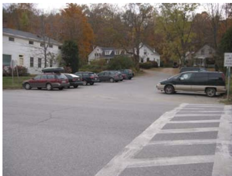
The Parsonage Lane-VT 100 intersection lacks definition. There is a continuous curb-cut along Parsonage Lane to the Village Grocery.
