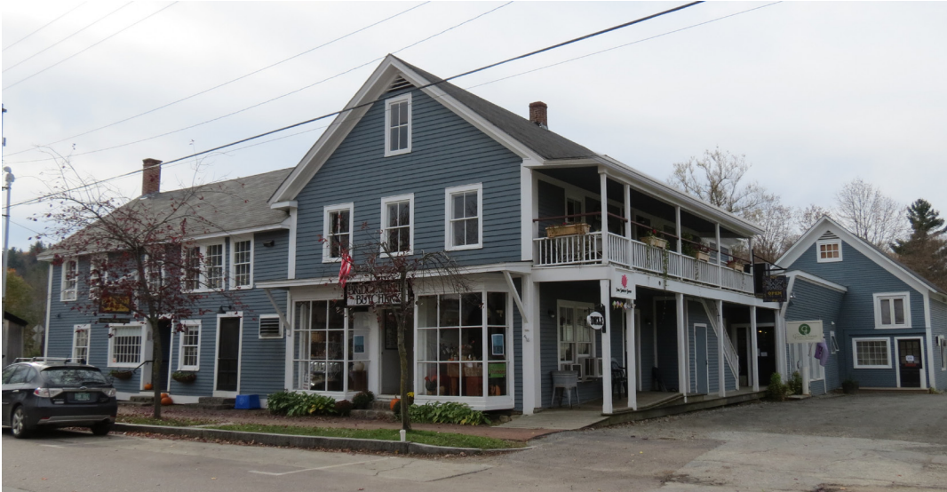
40 Bridge Street – Existing Façade Conditions
