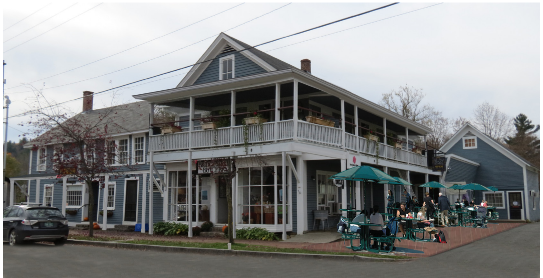
40 Bridge Street – The last step was to add posts to the front of the building.
