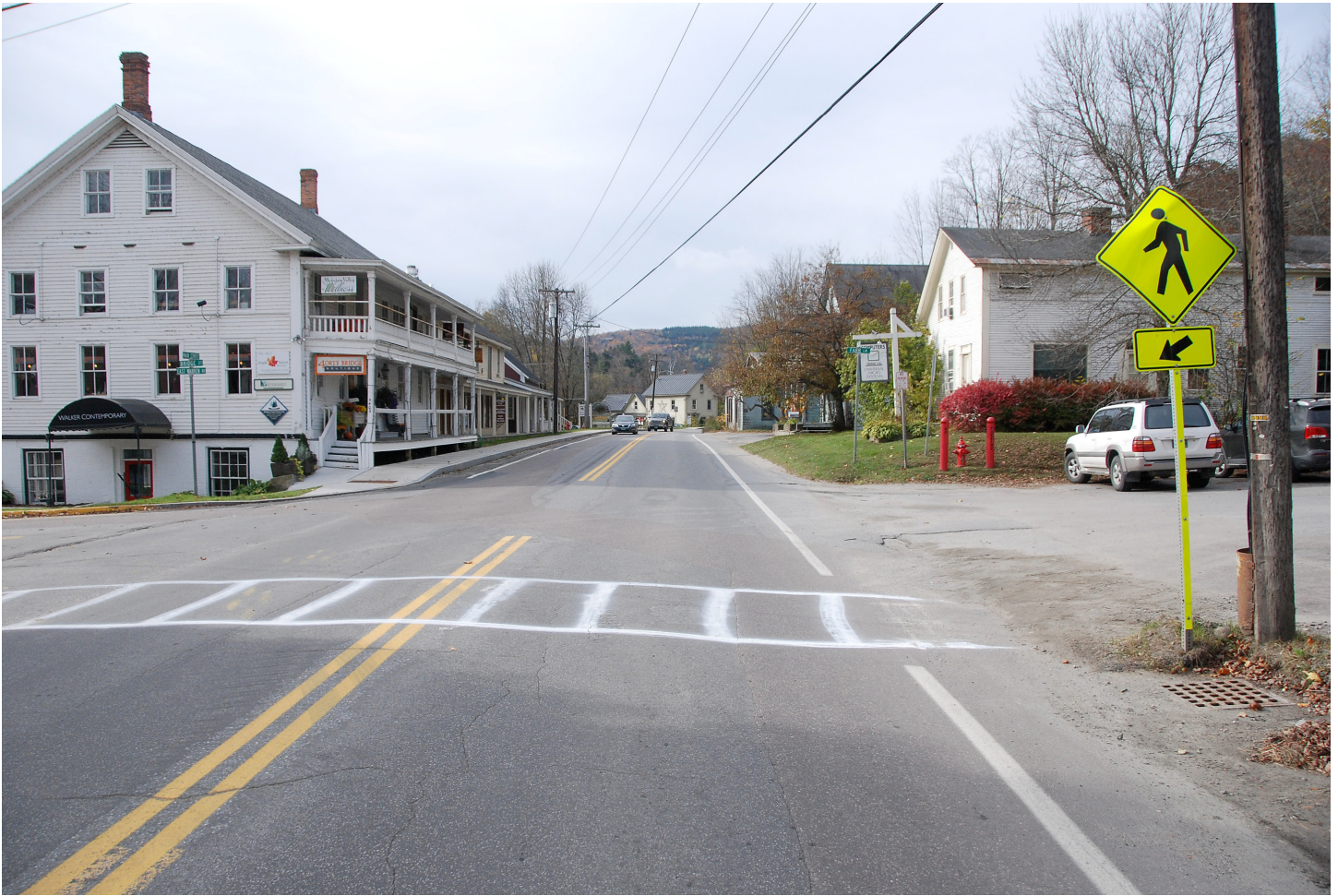
Main Street @ Bridge Street Intersection: Existing Conditions
