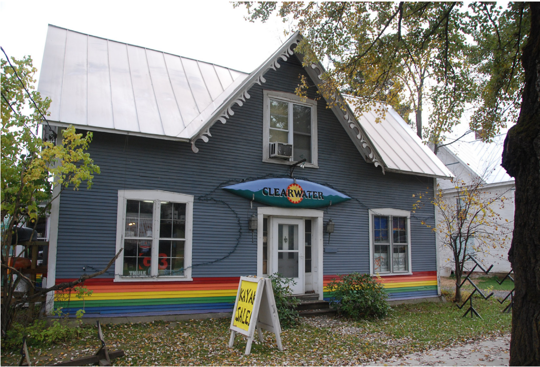
4147 Main Street – Existing Façade Conditions
