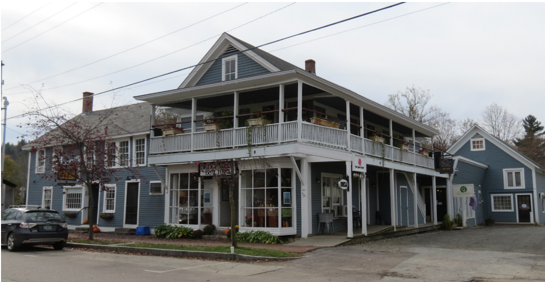
40 Bridge Street – The first step was to return the second floor porch to the front of the building.
