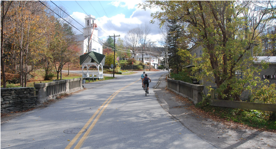
Village Bridge: Existing Conditions
