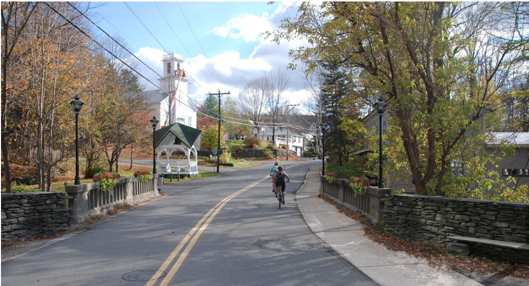
Village Bridge: Proposed Conditions
